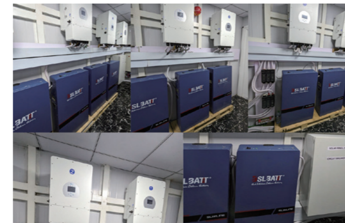
96kW Deye Inverter / 10*B-LFP48-300PW 153kWh / 120kWp Panel
