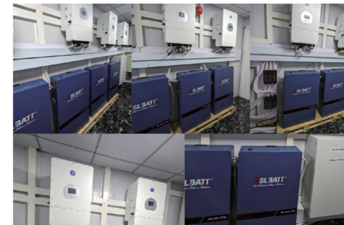
96kW Deye Inverter / 10*B-LFP48-300PW 153kWh / 120kWp Panel
